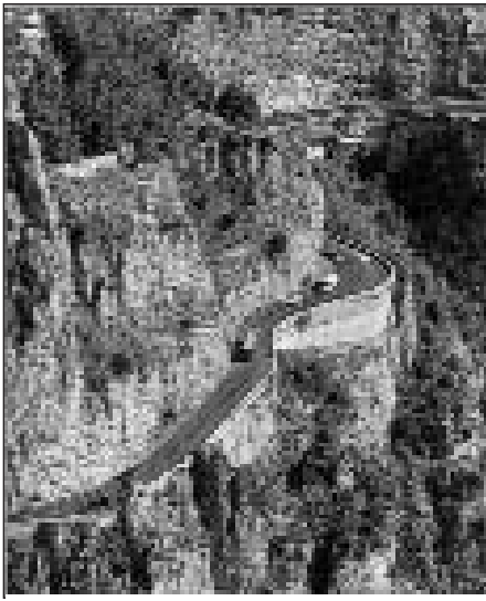
Building of the Amalfi Drive entailed some dramatic highway engineering with its retaining walls, cantilevered roadways from the sheer face of the mountains.
